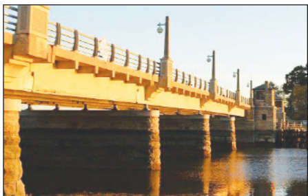
The Bayville Bridge
