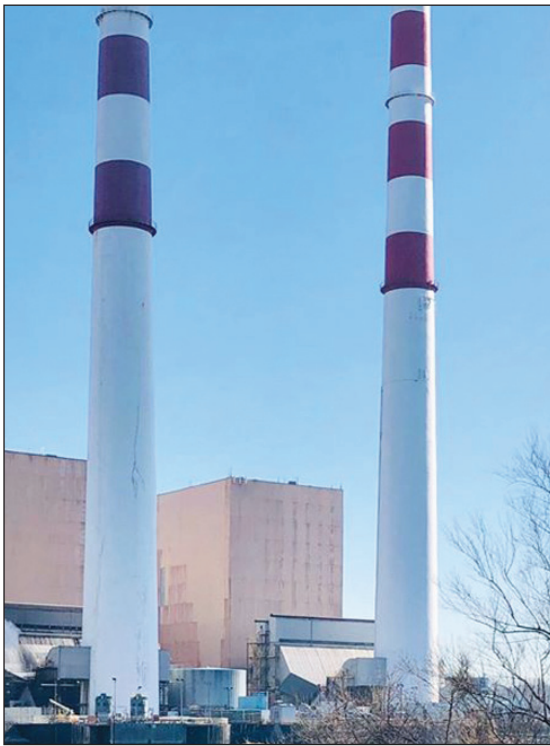
The Northport Power Plant
